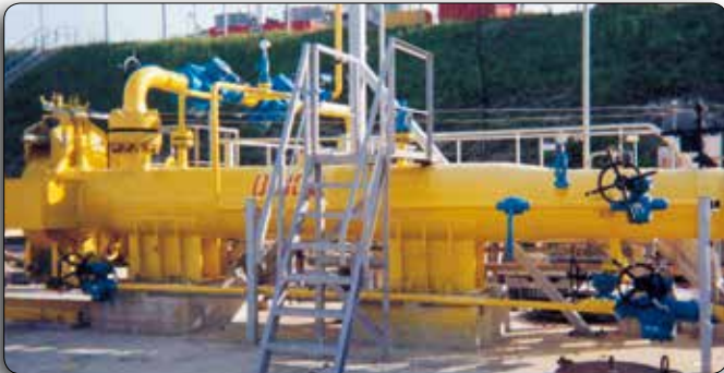
Client: SOFRESID SAIPEM France Location: Russia Pig Launcher "Beregovaya Compressor Station" Valves: DN 2" - 4" - 8" - ANSI 2500.
